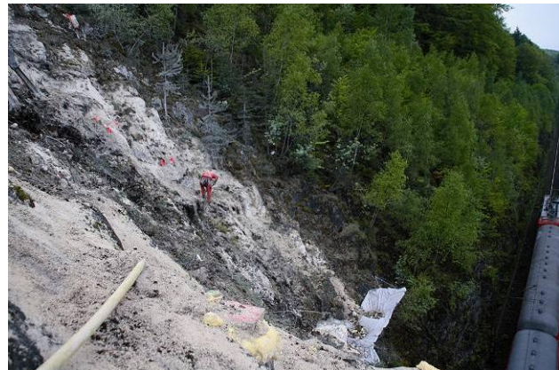
Preparation of protection against falling
