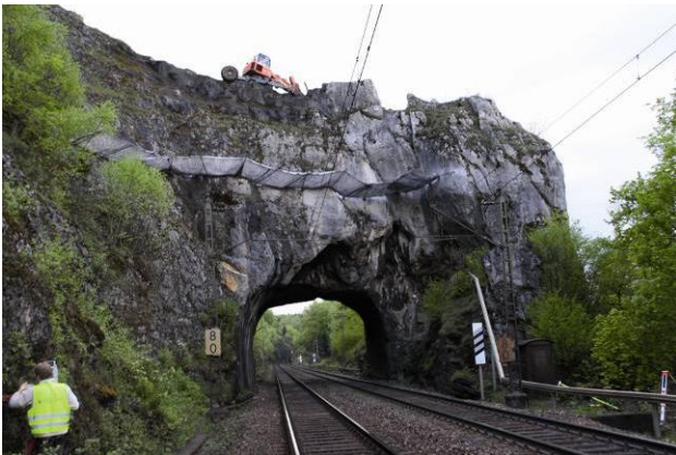
The 16 m rock tunnel
