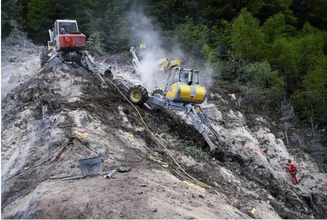
Drilling at 60° decliend slope
