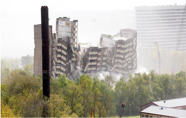
Blasting of the second tower block
