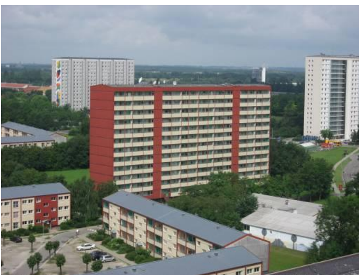
The 13 story Ruskær Building. Picture taken from South East. Free space to the West side of the building should be noticed.
