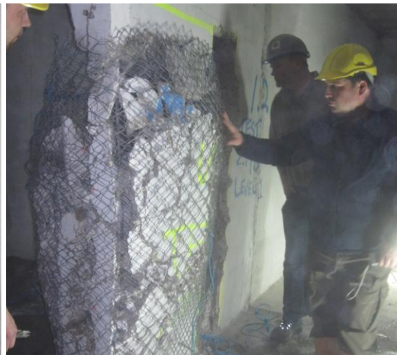
Result of test blasting.
