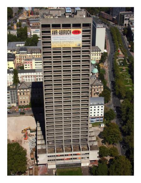
The basic principle of the blast demolition was a first vertical collapse of the skeleton part and a following folding of the core. The first vertical collapse was caused by blasting all columns in five floors. The three seconds later core folding completed the building drop down to an only 8 m high debris heap with a total length of about 100 m and a breadth of about 50 m.
