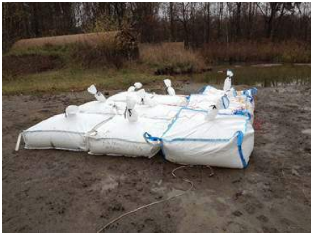
The 3 x 3 bag layout – side by side arrangement
