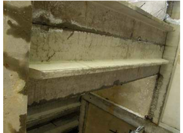
b) The bottom view of the girder before the test
