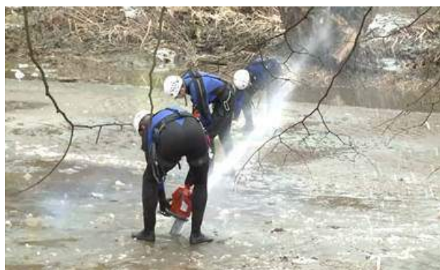
a) Preparation of holes for charge placement
