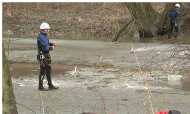
b) Placing of charges under the ice
