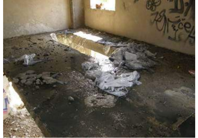
b) The floor perforation
