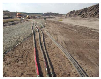
Blasting Pipe with up to 14 decks/charges - realized (Austin Powder)
