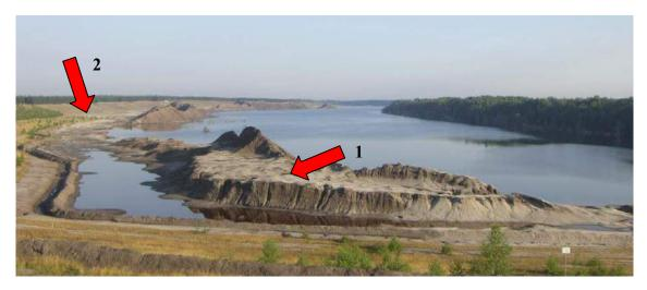
Mine dumps at the lake "Nordrandschlauch", decommisioned lignite mine Spreetal; Arrow 1 – loose mine dumps at the coast line Arrow 2 – improved slopes
