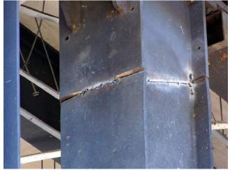
the application of 292 shock-tube detonators is not appropriate for such an operation. The tolerances of the delays may have led to the cut-offs.
