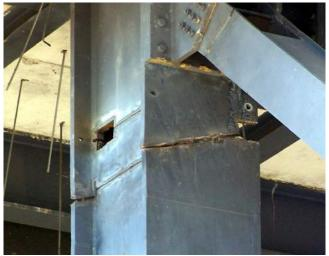
Fig. 5: improper cut
