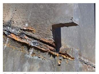
Fig. 7: insufficient cut after blast (attempt)
