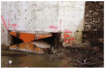
Fig. 9: steel hinge
