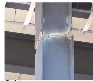
Fig. 6: improper cut
