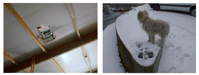
Example 2: Damage to a factory roof and blocks landing approximately 200 m in front of the blast
