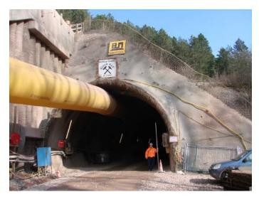
Fig. 2: West portal of the new Zierenberg Tunnel ('Monika Tunnel') alongside an embankment reinforced with bored piles
