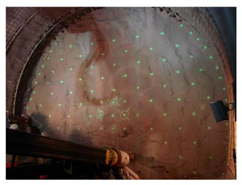
Fig. 16: Drill pattern on the reinforced tunnel face (roof section) marked by a laser theodolite
