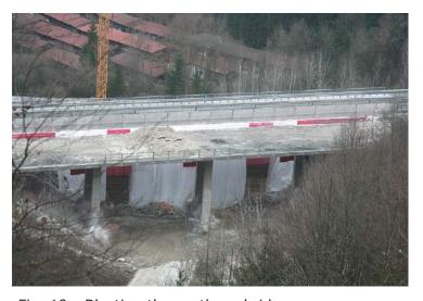
Fig. 10a. Blasting the northern bridge
