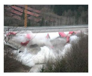
Fig. 10b - 10c. Blasting the northern bridge
