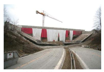
Fig. 11. Northern bridge, blast results
