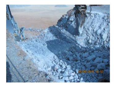
5.20 p.m. We designated the spot for placing the securing ropes. The channel was 2m in northerly direction from the edge and had the dimensions of 6.0 x 0.4 x 2.5m.
