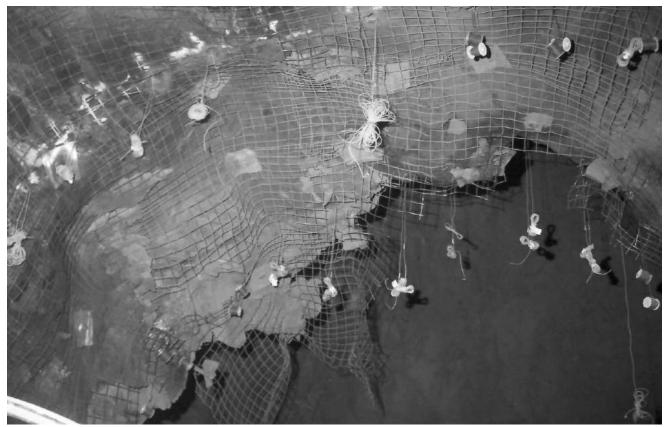
Figure 8. Charging complete for the hook-up process to tie it into the detonating cord at the open stope brow
