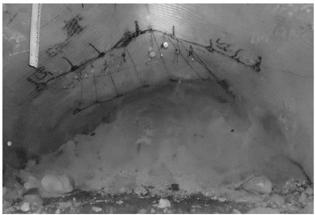
Figure 6. Hook-up for a single SLC ring with risks partially controlled with backfill, shotcrete and bunding
