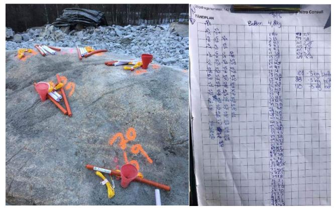
Figure 6.1 Left: The numbers of detonators for that hole together with the charge for lower deck. Right: The documented tie-up together with all charges for the blast
