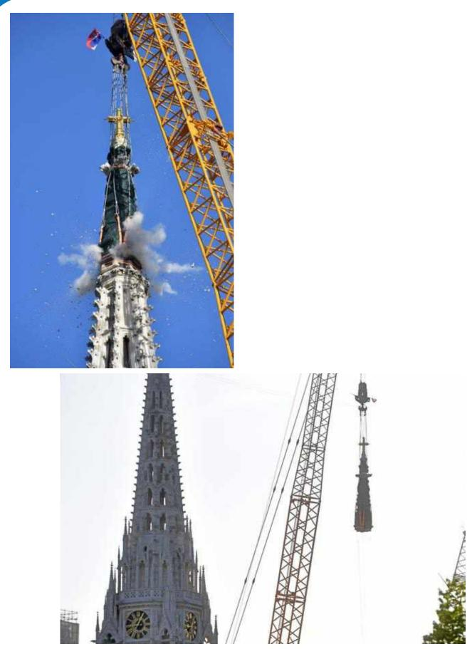
Figure 18. Blasting and lowering of northern tower (Photo: MORH/F. Klen)
