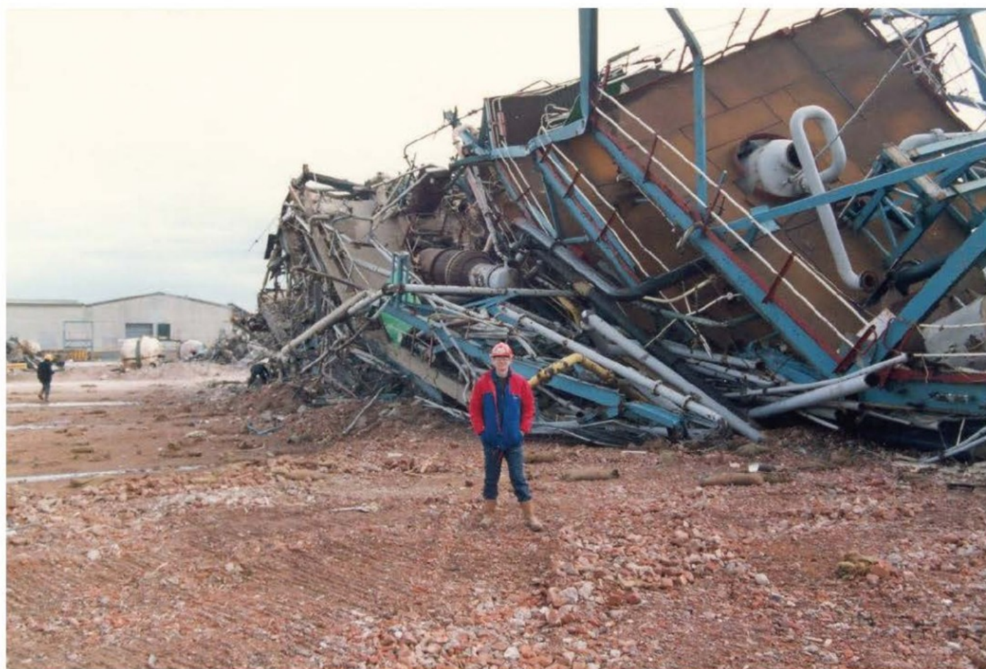
Author in front of demolished Paraquat tower
