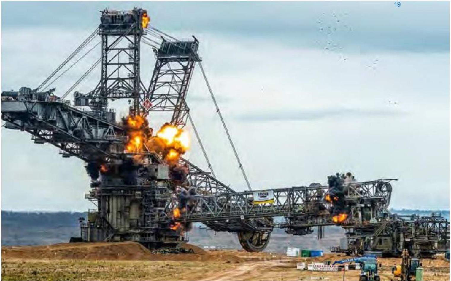
Fig. 6: Blasting of bucket-wheel excavator 259 | Photo: RWE (12 Demolition)
