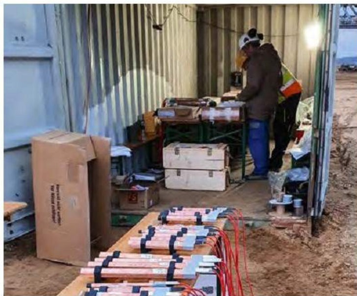
Fig. 4: Preparing the cutting charges for the steel structure lay-up work
