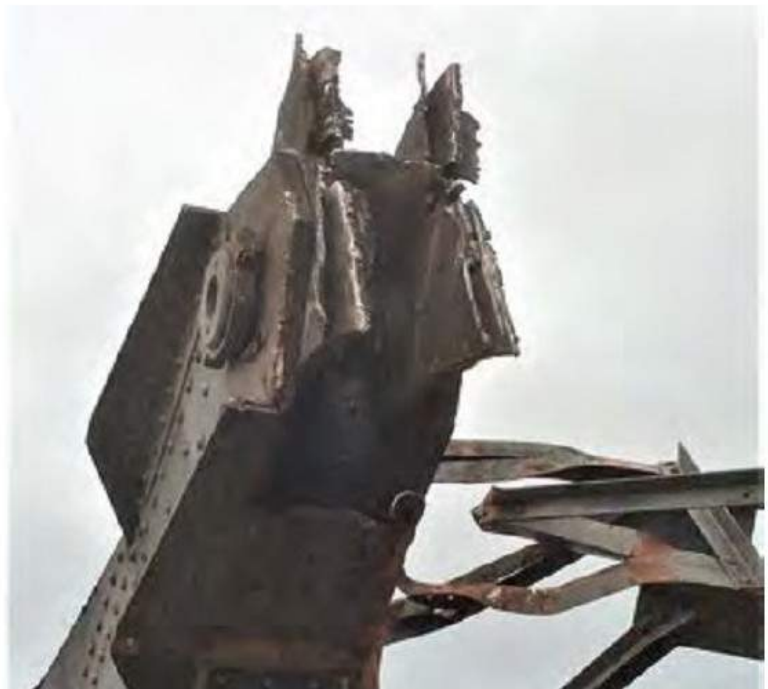
Fig. 7: Blasting result - multilayer sheet packs were completely cut through (13 Demolition)
