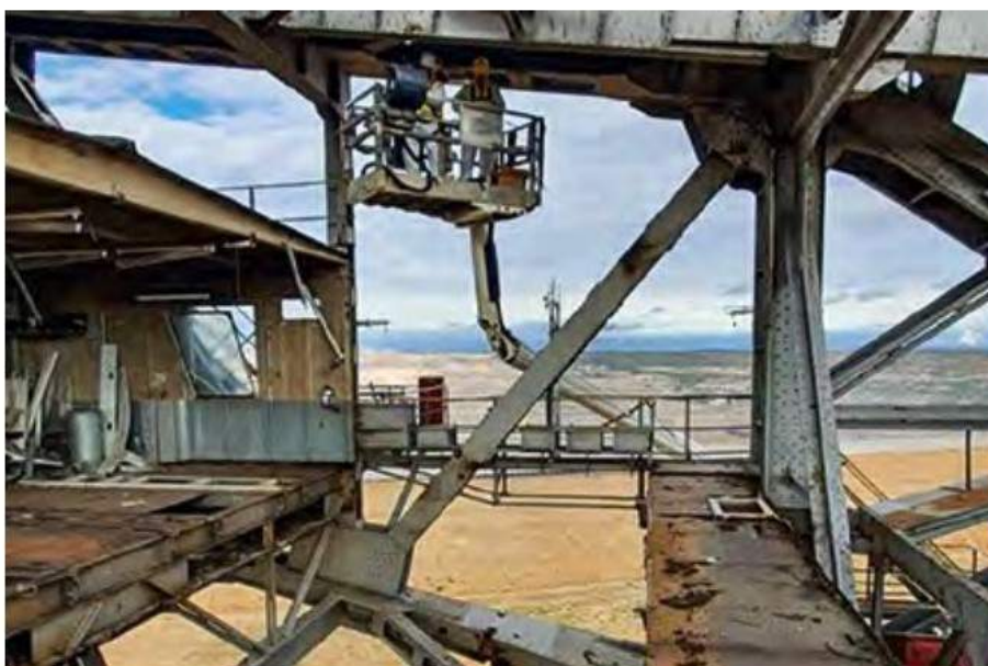
Fig. 5: Attachment of the cutting charges utilizing lifting platforms
