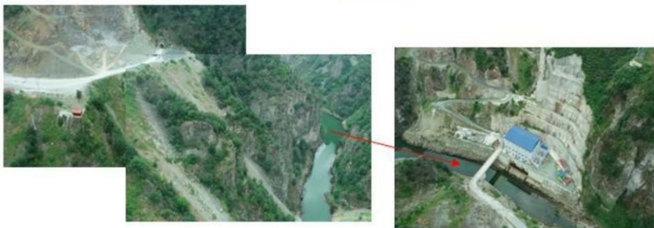
Figure 1-b) Drone photo showing quarry, valley, river, Darıca-2 HEPP location
