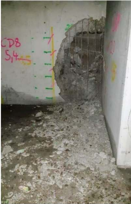
Fig. 6: Blasting result borehole charges Photo: Thüringer Sprenggesellschaft mbH
