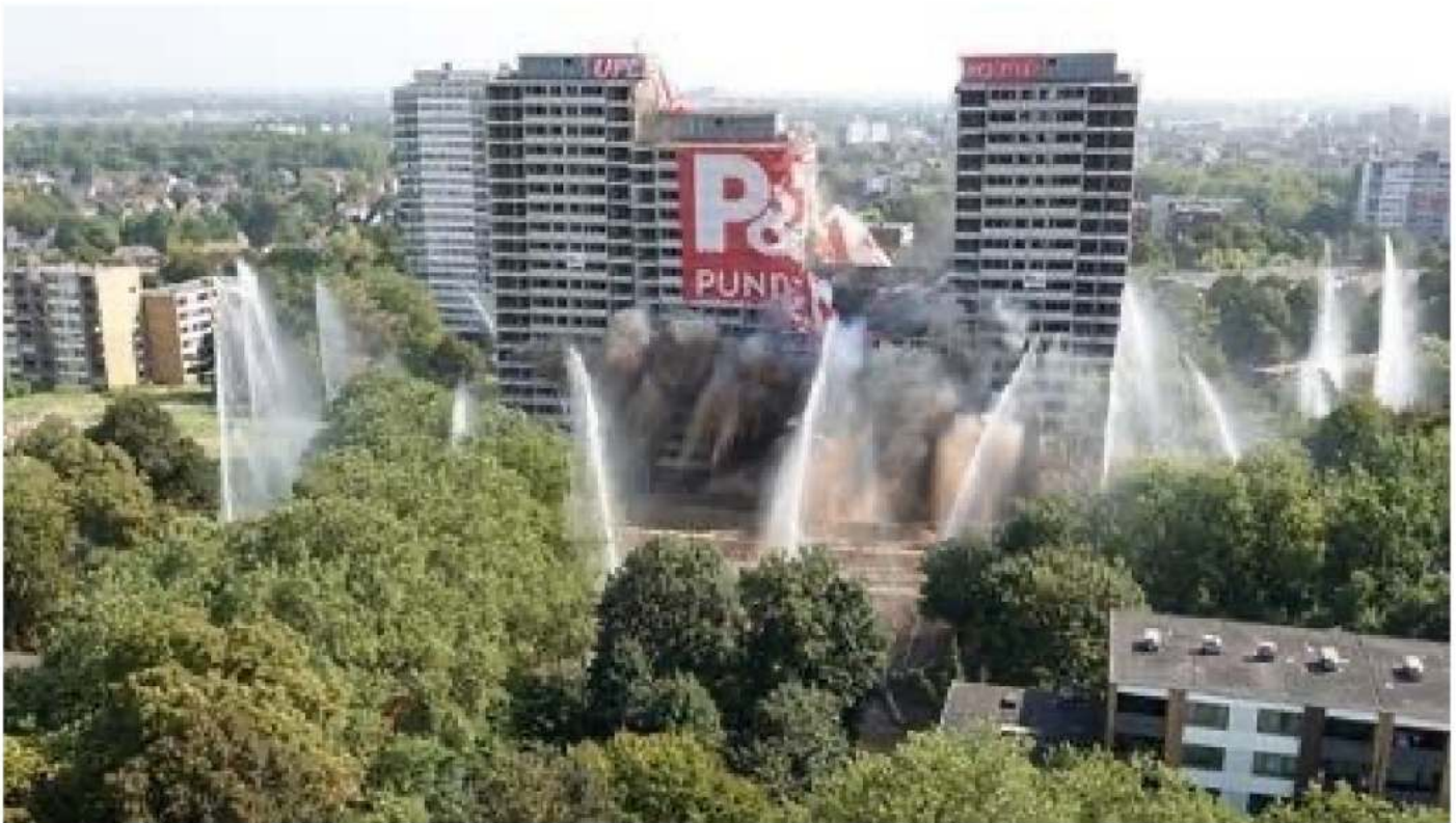
Fig. 11: Blasting, photo: Mobile Image and Measurement Service Michael Böhme
