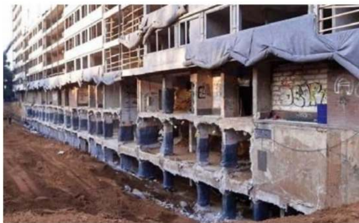
Fig. 10: Preparing safety measures Photo: Thüringer Sprenggesellschaft mbH
