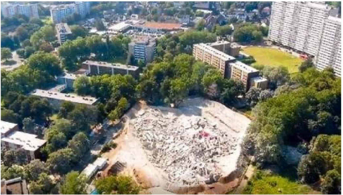
Fig. 12: Blasting result, photo: rebuild.ing GmbH
