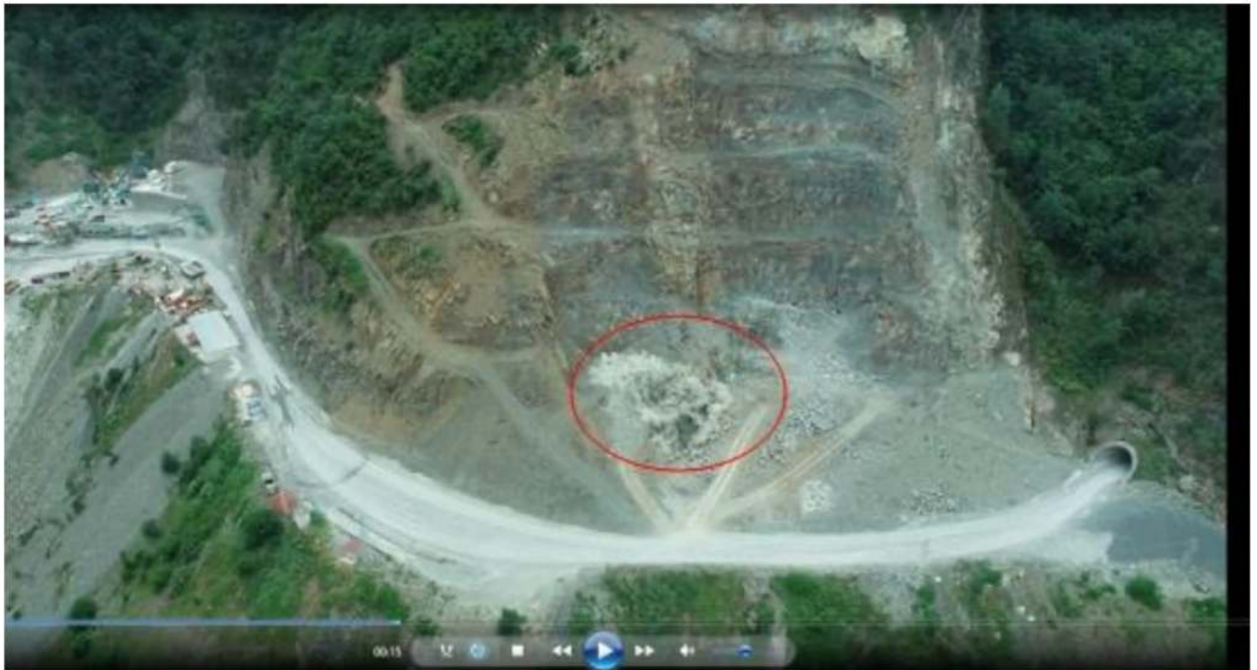
Figure 7. Blasting Image Performed With Electronic Ignition
