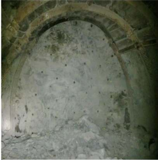
Fig. 7 Transverse gallery in rock face, before and after blasting
