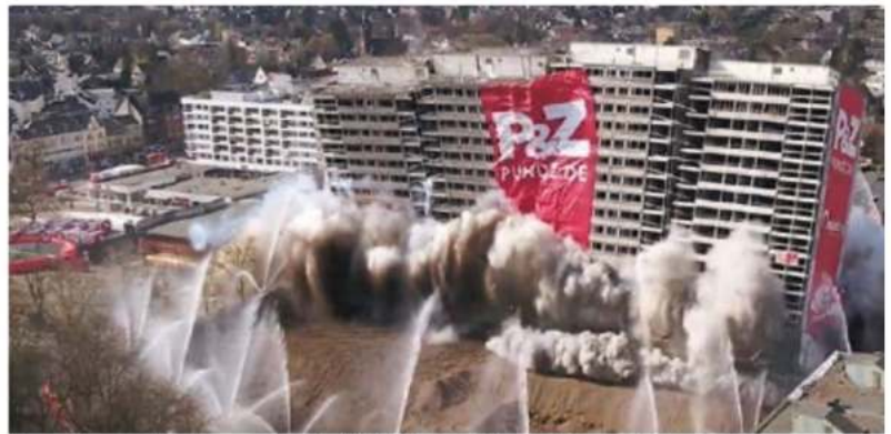
Fig. 1: Blasting first "White Giant", photo: rebuild.ing GmbH
