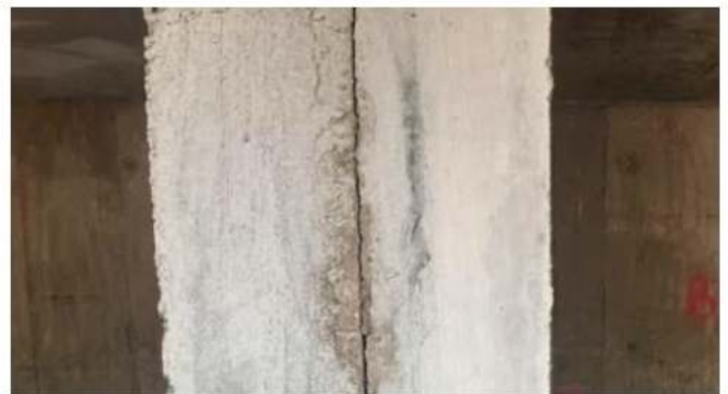
Fig. 3: Joint wall, Photo: Thüringer
